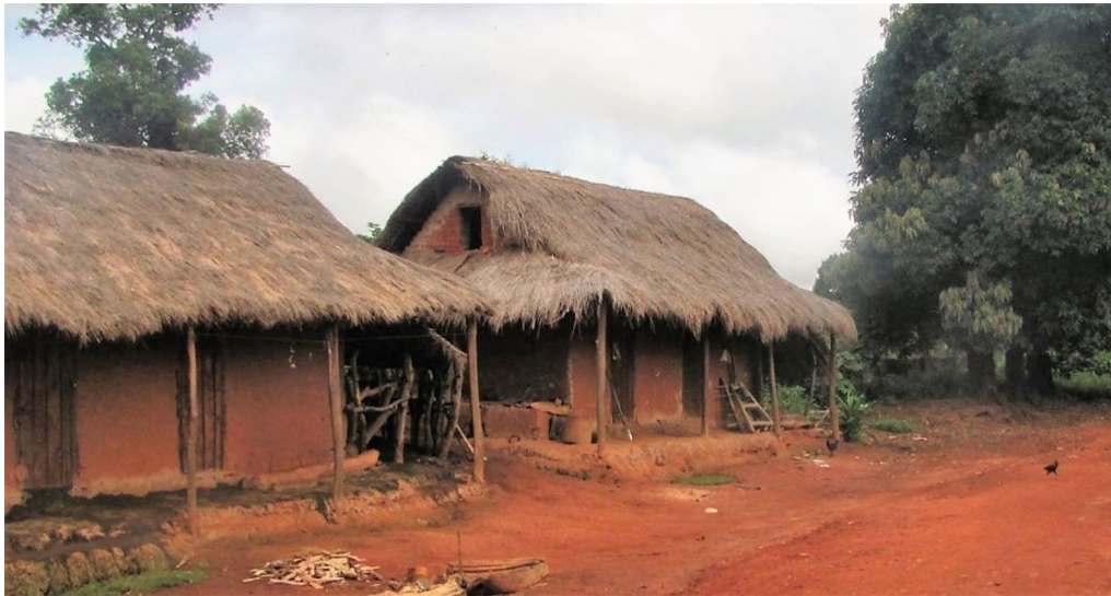
Fig. 2 Typical Malagasy houses in Andriba rural area. The houses are built with adobe walls and thatched roofs, and usually composed of one or two rooms. The picture was taken in the village of Ambohitromby located in the rural commune of Andriba, Madagascar
